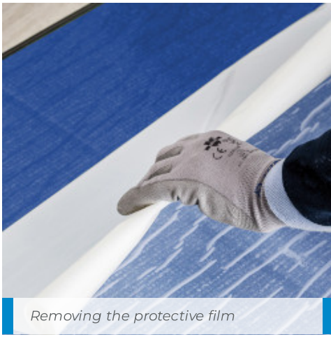
Installing self-laying LVT flooring on the adhesive film
