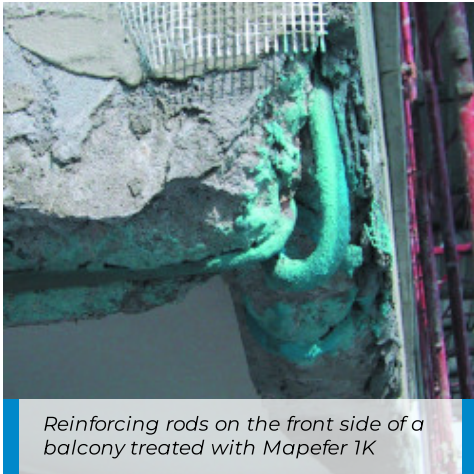
Demolition of degraded concrete
