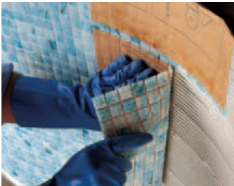
Glass mosaic 2x2 cm installation in a swimming pool with Adesilex P10 mixed with Isolastic diluted 1:1
