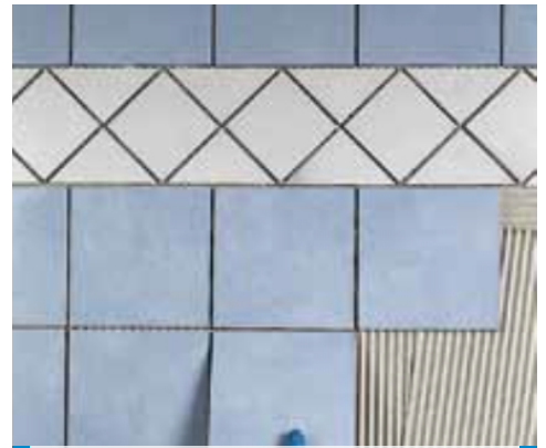
Installation of single-fired tile on gypsum board wall
