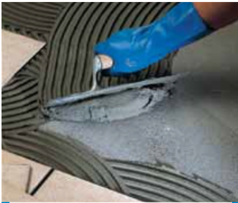
Installation of single-fired tile on floor
