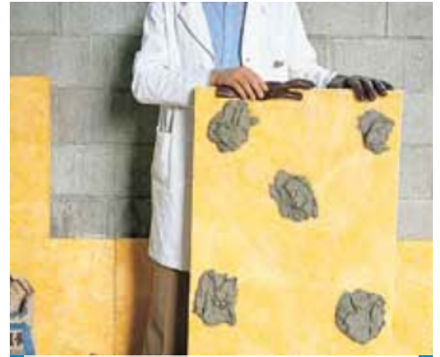
Spot-bonding insulating panels on untreated wall
