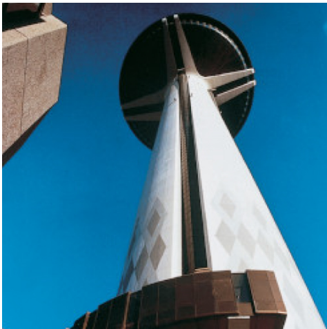
An example of an installation of clinker on concrete with Kerabond + Isolastic - New Telecommunication Tower - Kuwait City (Kuwait)
