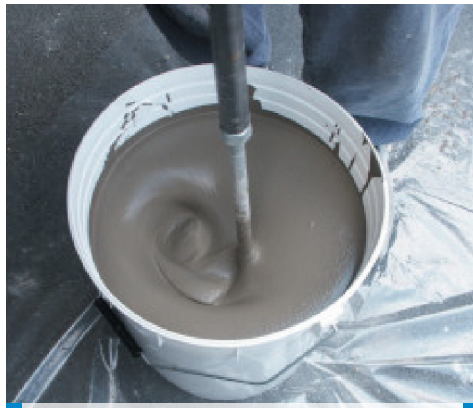
Preparation of the product with a drill
