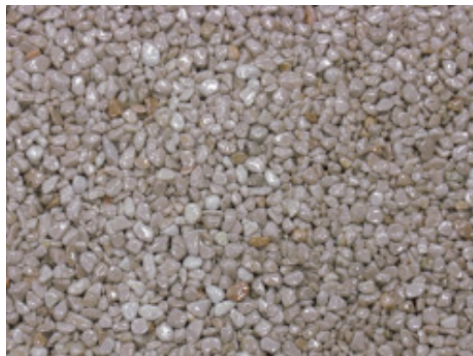
Application of the mixture of natural aggregates + Mapefloor I 910
