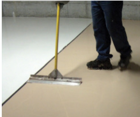
Smoothing Ultratop immediately after spreading
