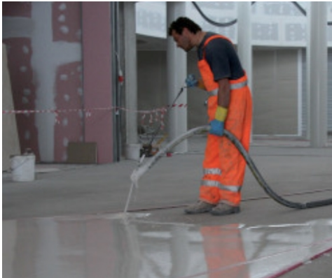
Mechanical application of Ultratop
