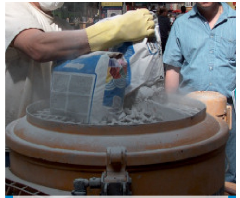
Preparation of Ultratop in a mixer
