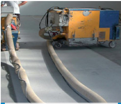
Preparation of the substrate by shot-blasting
