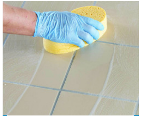
Cleaning and finishing joints with a hard cellulose sponge
