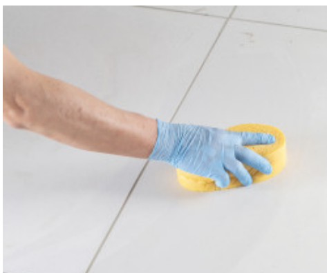
Cleaning and finishing the joints with a hard cellulose sponge
