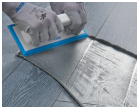
Spreading Ultracolor Plus on wood-effect porcelain floor tiles with a rubber float
