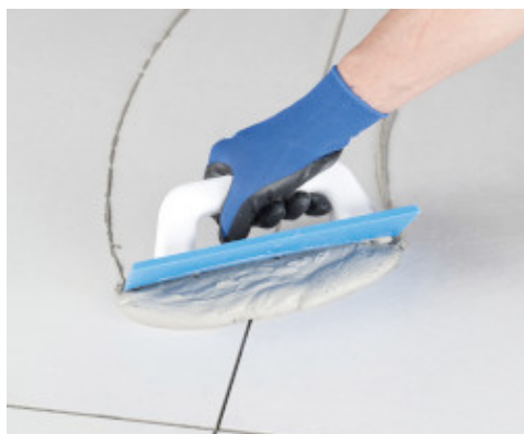
Spreading Ultracolor Plus on porcelain floor tiles with a rubber float
