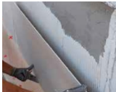
Applying a thin porcelain tile on an external façade
