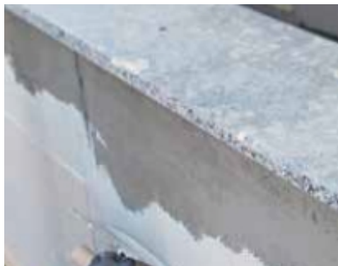
Laying on an external façade: application of adhesive on the substrate
