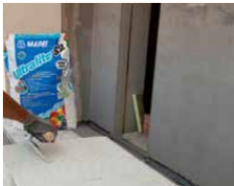
Spreading the adhesive on the back face of the tile
