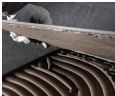
Installing thin porcelain tile on floor
