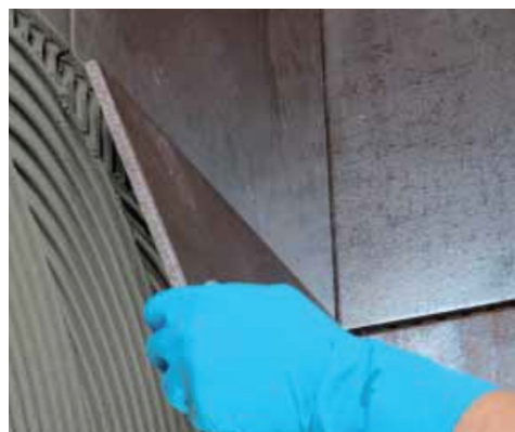
Laying large-sized tiles on walls
