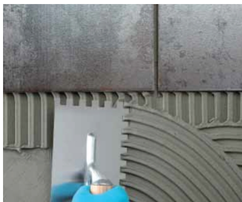
Spreading Ultralite S1 with a notched trowel on wall
