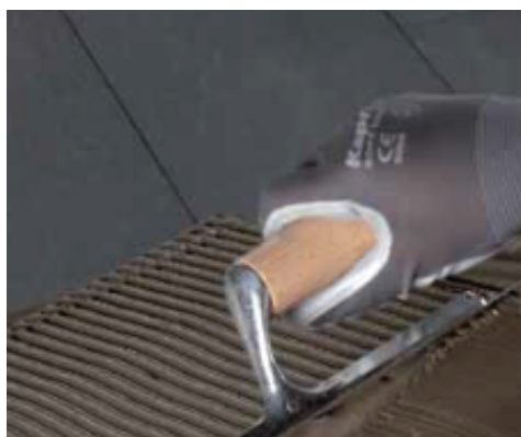
Spreading the adhesive on the back of the tile
