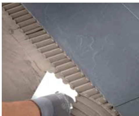
Spreading the adhesive on floor with a 9 mm round-tooth notched trowel
