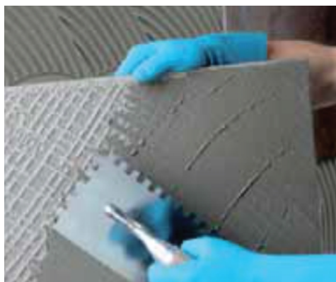
Spreading adhesive on the back of the tile
