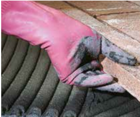
Installation of hand made terracotta on an uneven substrate
