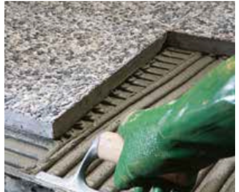
External installation of relief terrazzo "graniglie" tiles
