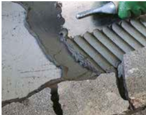
Installation of external hewn back stones with or without buttering, depending on thickness and size
