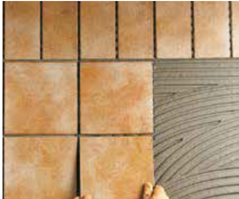
External installation of clinker tiles
