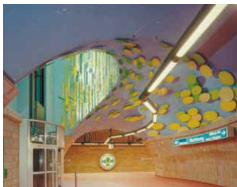
An example of an installation of granite with Granirapid Subway in Mulheim Ruhr (Germany)
