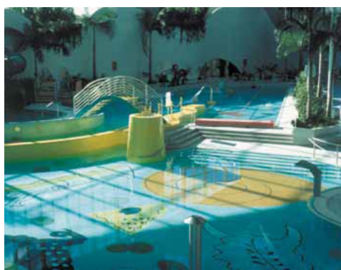
An example of mosaic and klinker installed in a swimming pool
