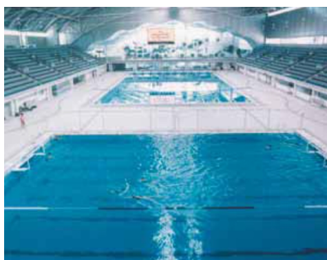
An example of mosaic and klinker installed in a swimming pool - Olympic Centre, Sydney (Australia)
