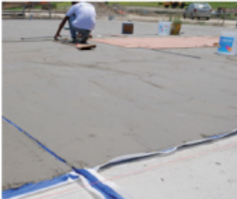
Waterproofing screeds with Mapelastic and Mapeband
