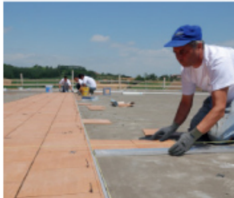
Installing ceramic with Kerabond T + Isolastic
