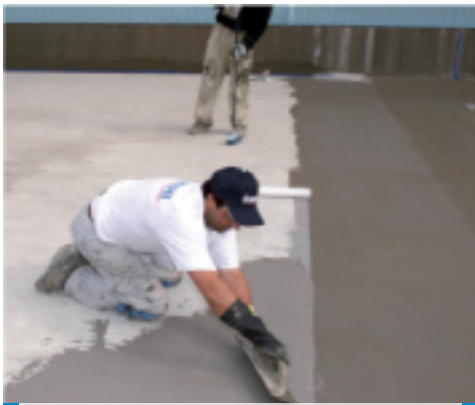
Waterproofing a swimming pool with Mapelastic
