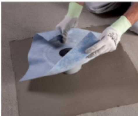
Application of Drain Vertical on Mapelastic
